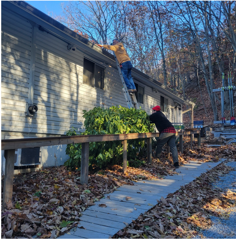
House Director Kevin Broderick and Justin Siris cleaning the gutters!
